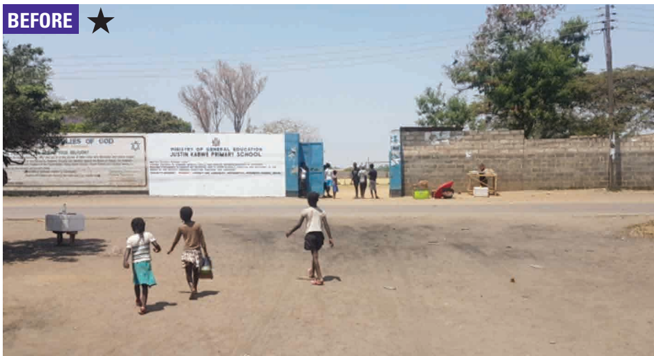
Before intervention: SR4S assessed the school entrance as a dangerous 1-star for safety. Justin Kabwe primary school in Lusaka, Zambia before infrastructure improvements.
