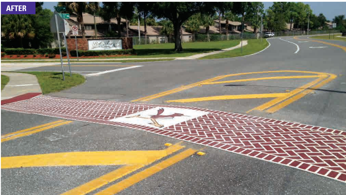
Safe School Zone upgrade in Seminole County, Florida
